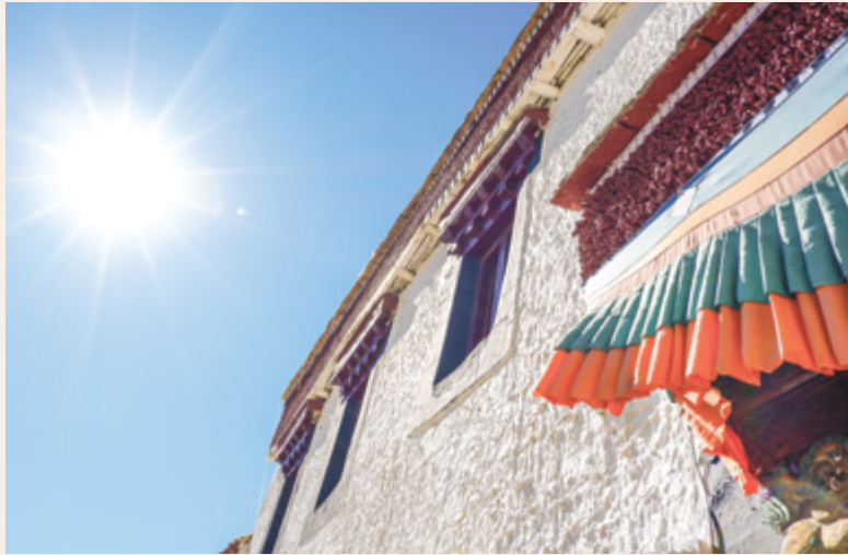
A typical monastery wall and roof
